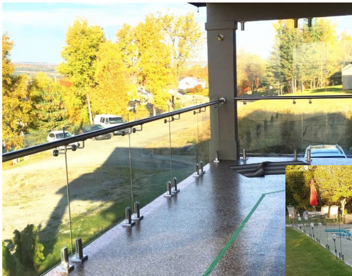
Type 4 : Glass railing with glass spigots
