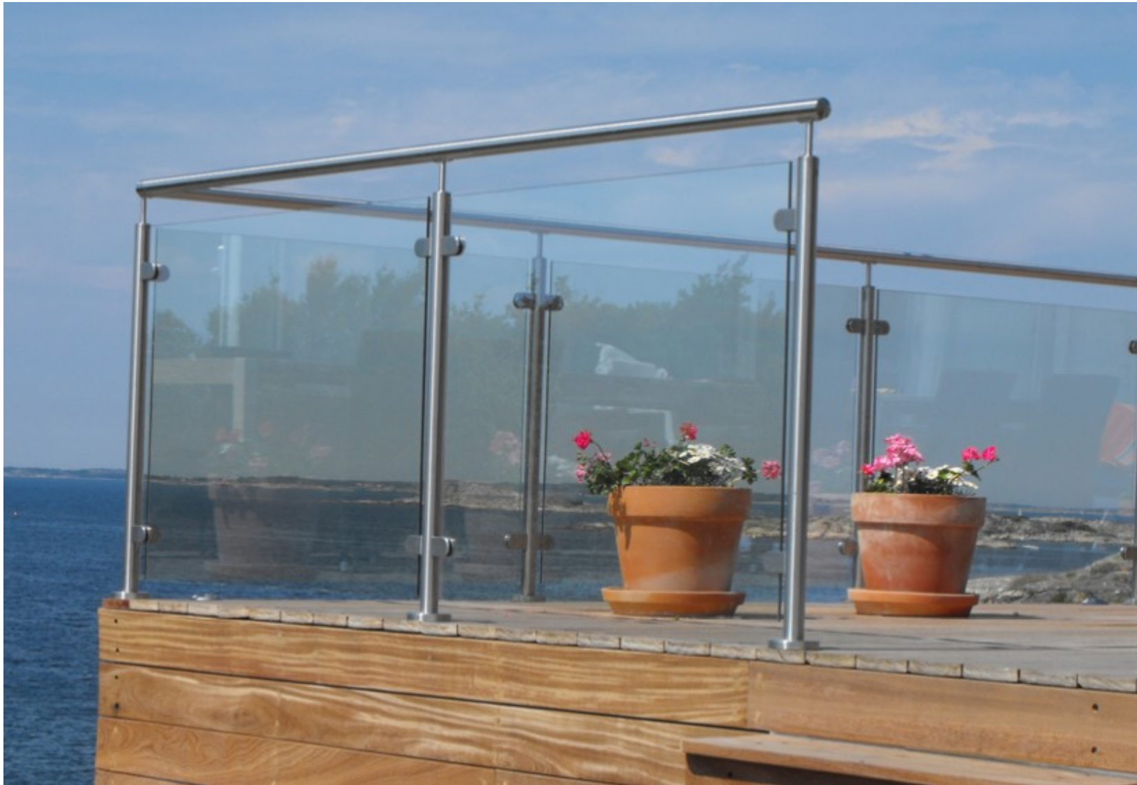
Type 1 : Glass railing with stainless steel posts
